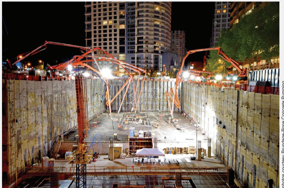
photos courtesy Brundage-Bone Concrete Pumping
