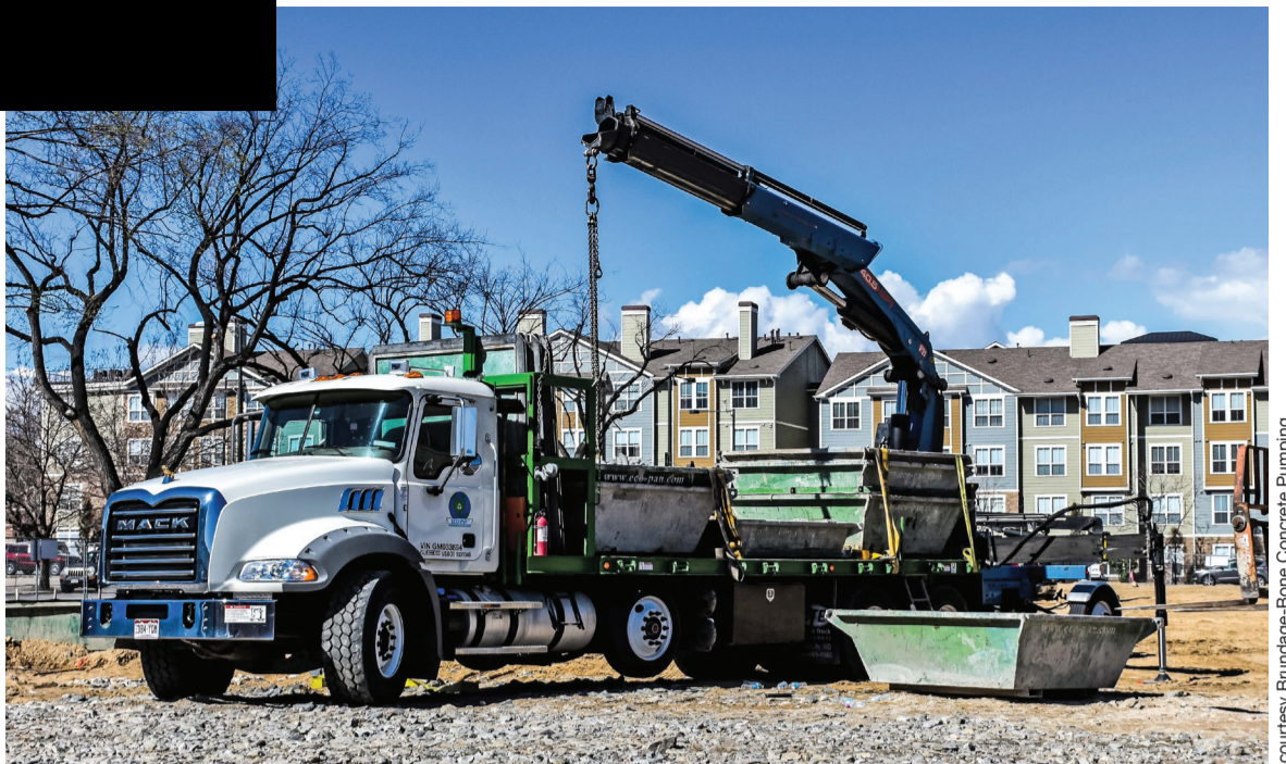
courtesy Brundage-Bone Concrete Pumping
